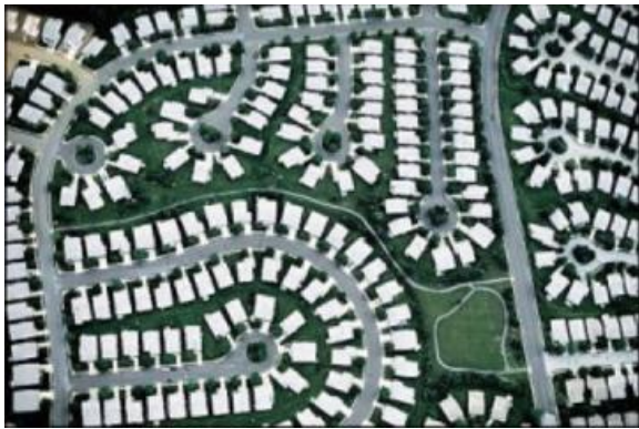
Residential development characteristic of suburban sprawl—similar houses situated on cul-de-sacs.
